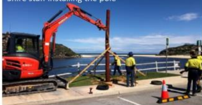
Shire staff installing the pole
